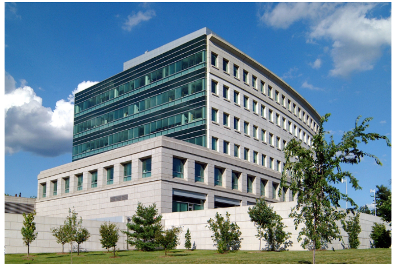
Natcher Conference Center (Building 45), National Institutes of Health (NIH)
